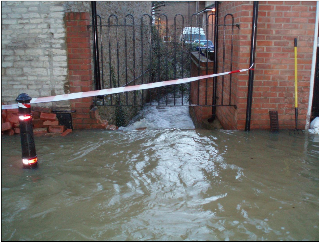
Figure 7: Section of wall removed on south side of Causeway by Oxfordshire Fire and Rescue Service to allow flood water to return to Back Brook
