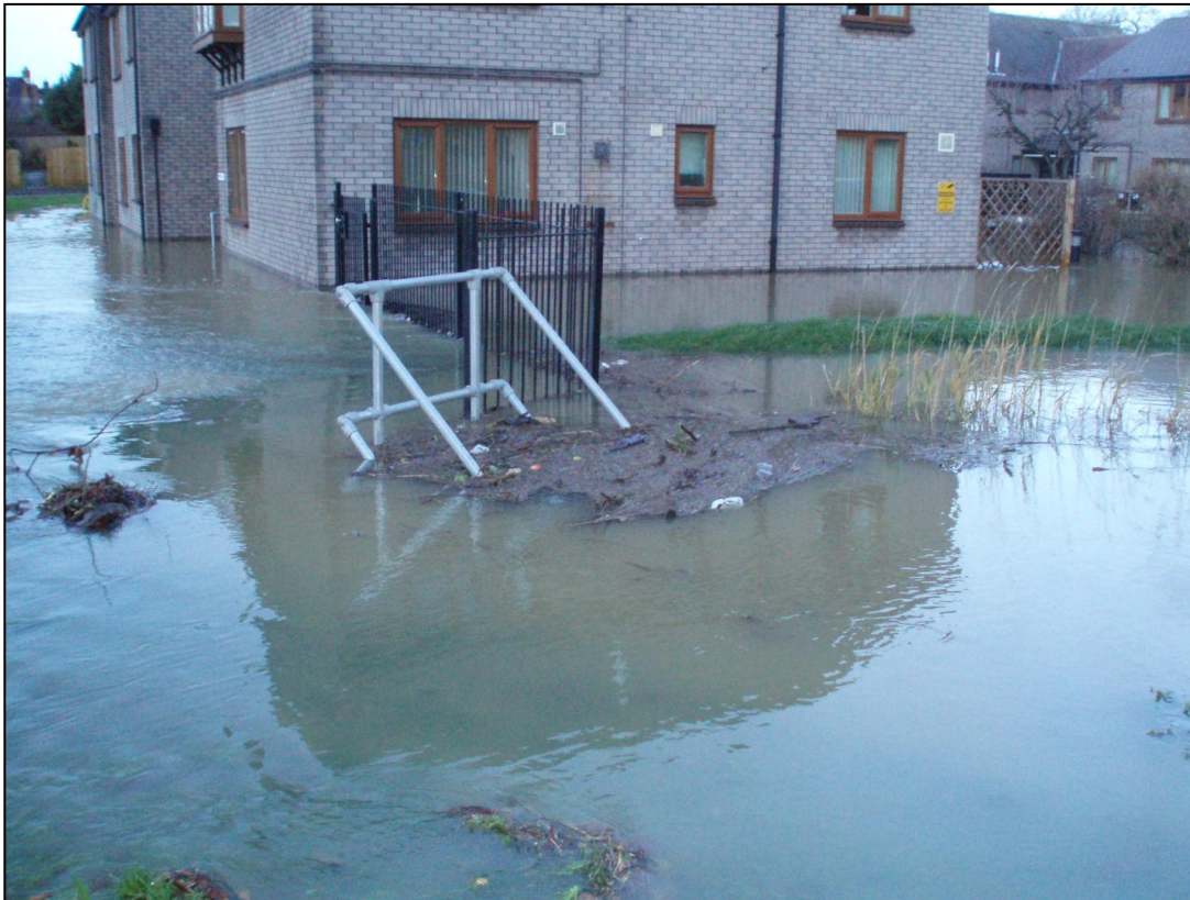
Figure 8: Guard rail of Back Stream culvert headwall surrounded by flood water
